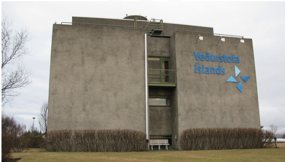
Figure 6: The Icelandic Meteorological Office Photo of the Icelandic Meteorological Office building (Icelandic Meteorological Office, n.d.)
