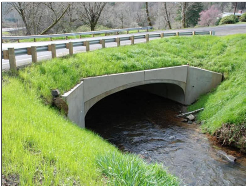
Figure 5.2: Example of a finished B-Series® buried bridge, a similar Contech® structure with different span and rise options (ArchiExpo, 2017)
