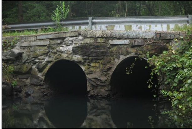
Figure 4.1: A downstream view of the existing culverts
