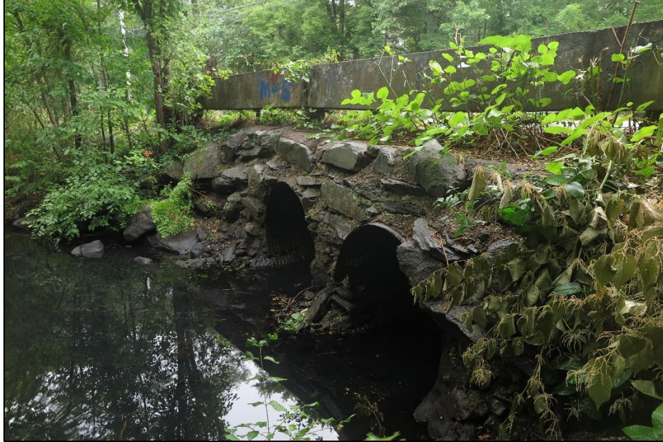
Figure 2.1: The inlet of the Walker Street stream crossing
