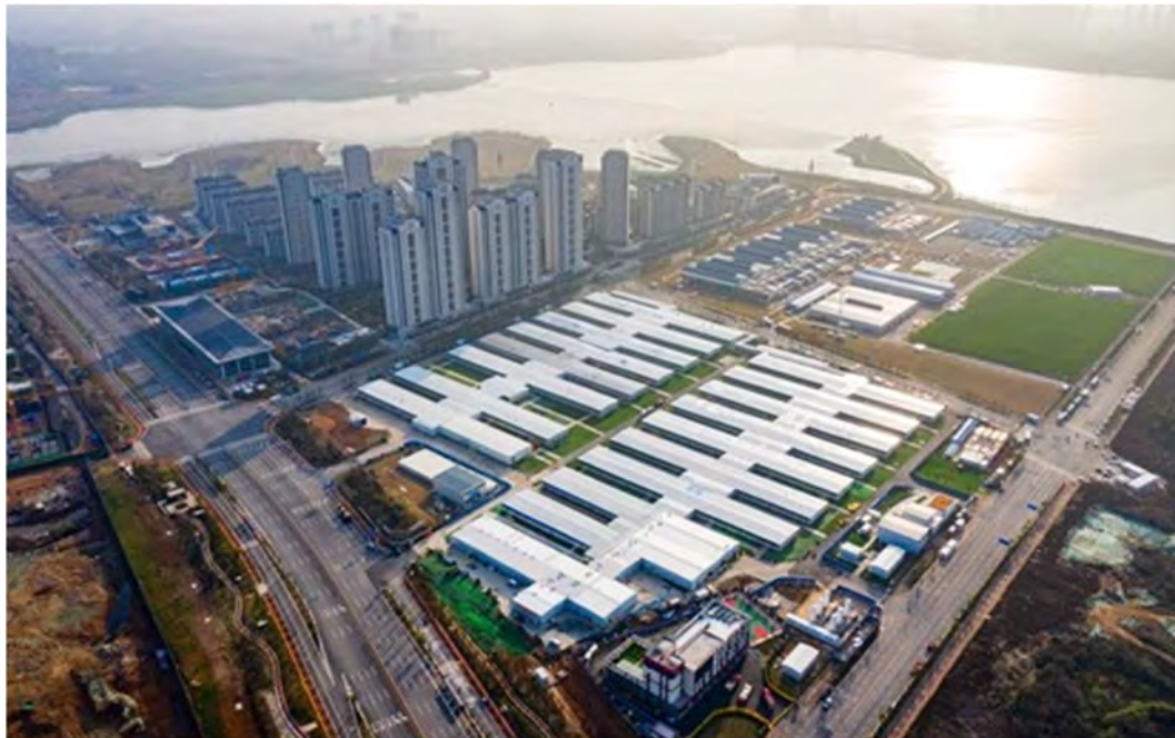
Figure 3: Huoshenshan Hospital (Mo, 2020)
