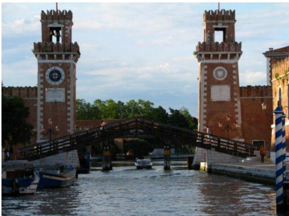
Figure 35: The Gates of Arsenal
