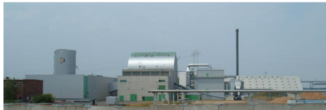
Figure 19: Masnedø CHP Power Station in Denmark
