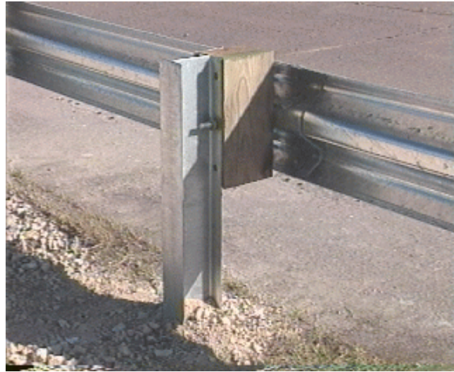
Figure 4.3: Modified G4(1S) with routed wood blockouts.(57)
