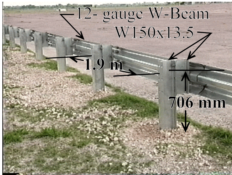
Figure 4.1: G4(1S) guardrail system.(56)
