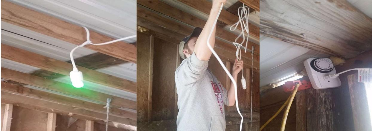
**Figure 19: The LED light (left), students install the light (center) and timer (right)**
