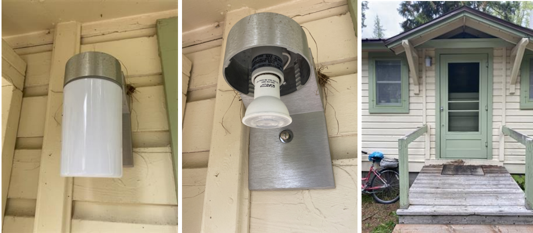
Examples of pictures of light fixtures, displaying a close up of the fixture (left); one a closeup of the bulb (center); and the fixture and its task area (right).
