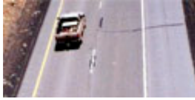
Figure 5-8: RMA roadway (Recycle Ohio, 2005)
