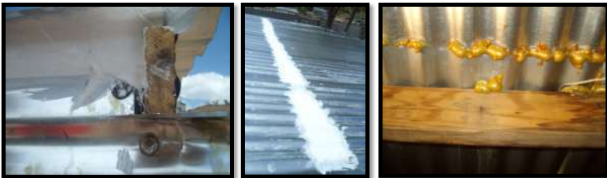
FIGURE 15: MULTIPLE WATERPROOFING TECHNIQUES 67
