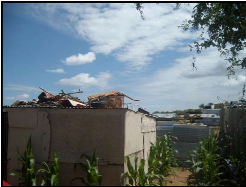
Holding roof down with found items.
