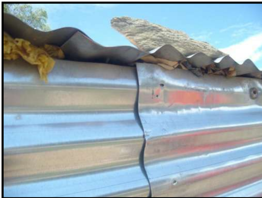
Blocking gaps from wind and rain.
