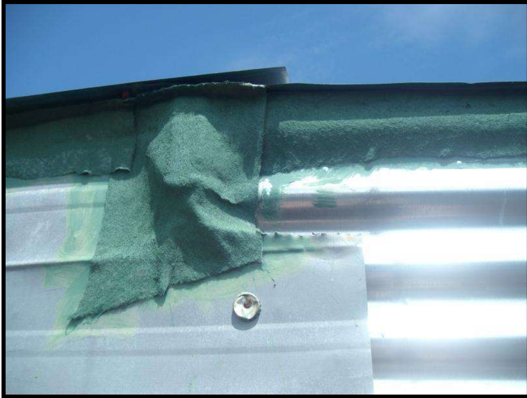
Waterproof sealant for leaks
