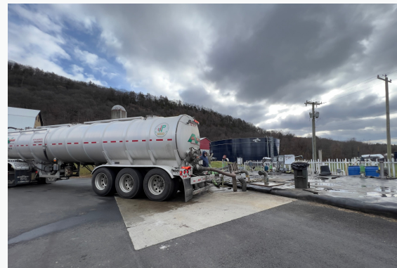
Figure 14: Anaerobic Digester and Transport Truck at Barstow's Longview Farm
