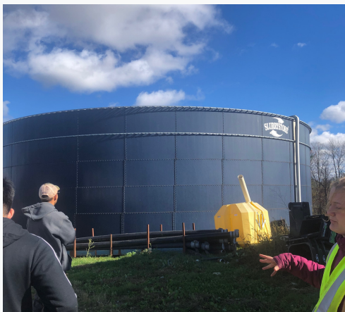
Figure 15: Anaerobic Digester at Jordan Dairy Farm in Rutland, Massachusetts
