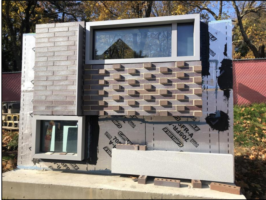
Figure 5.6: Current brick façade with two masonry velours
