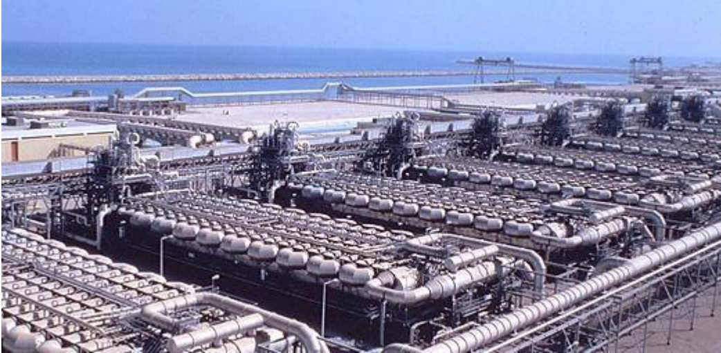
Figure 6: Multi-stage flash plant, Saline Water Conservation Corp. Al Jubail, Phase II Saudi Arabia (Sasakura Engineering Co., LTD)
