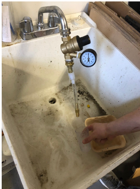
Figure 55: Basic testing of the water pressure regulator with one of the cups
