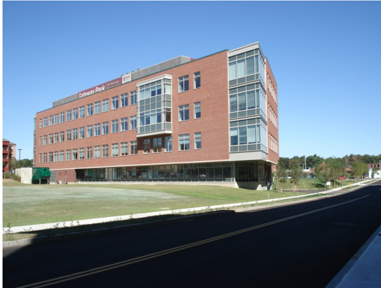
Figure 1: Side View of the Main and First Constructed Building at 60-68 Prescott Street
