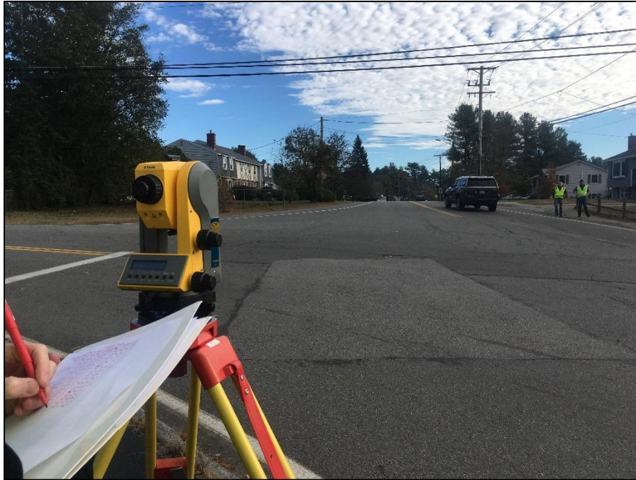
Figure 10: Surveying Equipment Set Up
