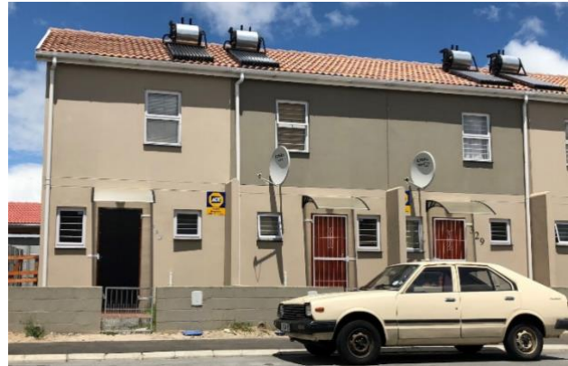
Figure 10: Some two-story RDP homes in Pelican Park in the Western Cape.
