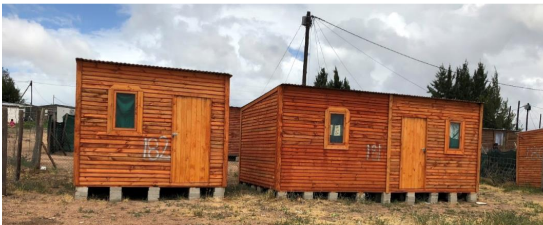
Figure 3: Some temporary houses, often referred to as Wendy homes, found in the TRA of Jamestown, Mountain View in the Western Cape.
