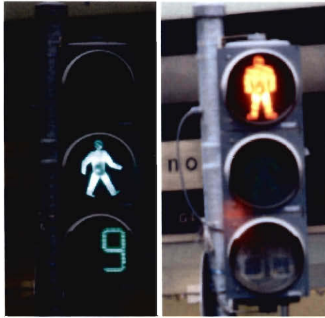
Figure 2.4: Pedestrian Crosswalk Warning System
