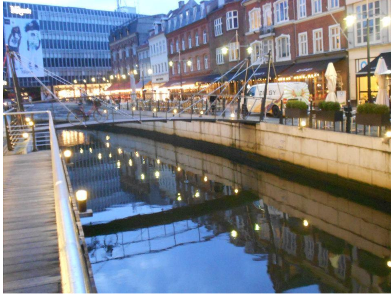
Figure 88: Aarhus Pedestrian Bridge 2
