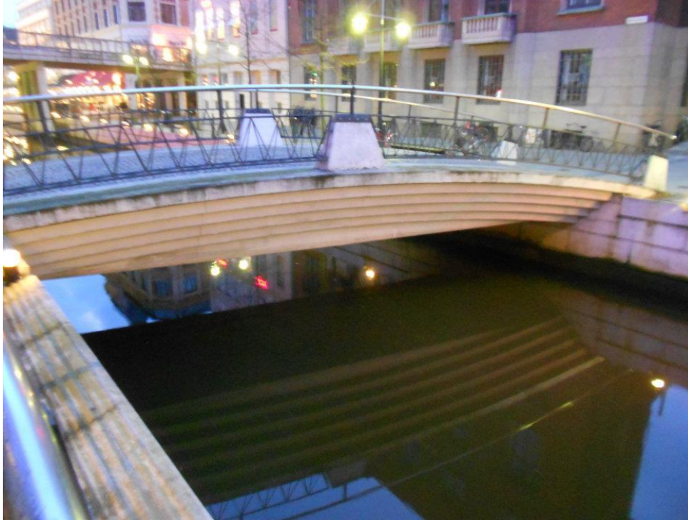
Figure 93: Aarhus Pedestrian Bridge 3
