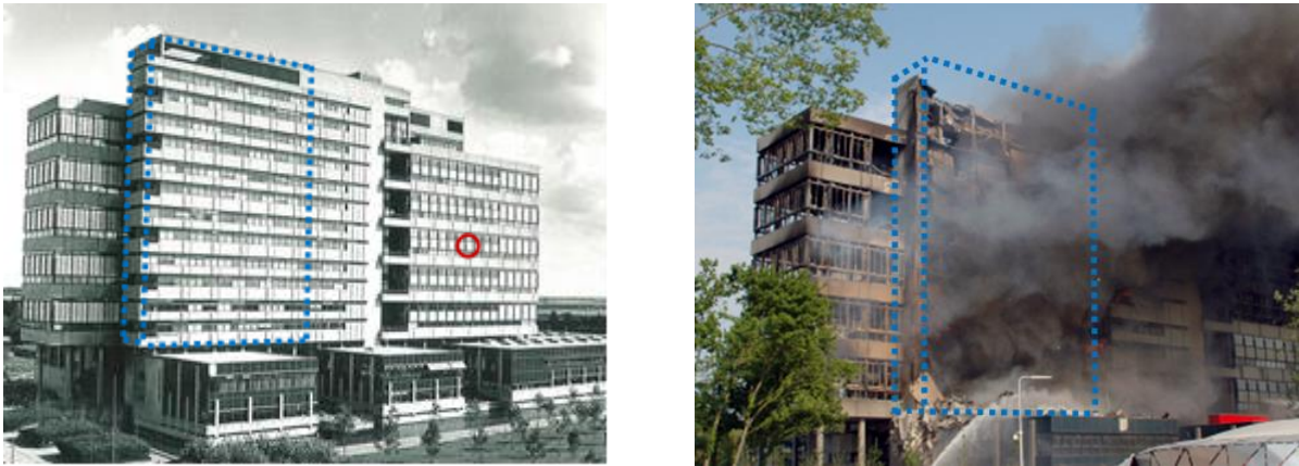
Figure 5. Fire origin (red circle) and collapsed portion of the building (blue dotted lines)
