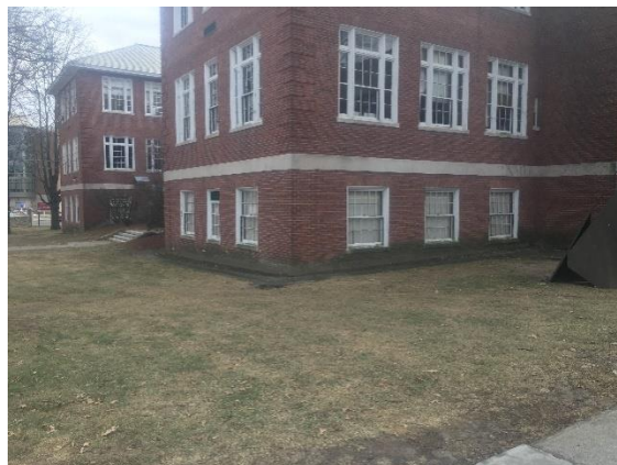
Figure 3: Exterior Grading of Existing Building
