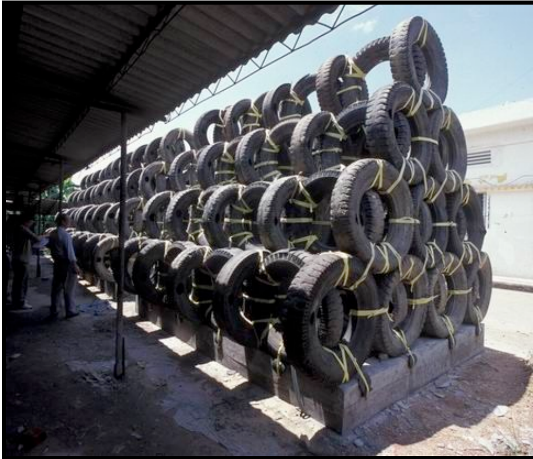
Figure 9 - A tyre reef unit prior to submersion, showing the nylon straps and base. Photo courtesy of Eric Yau (See Appendix I).
