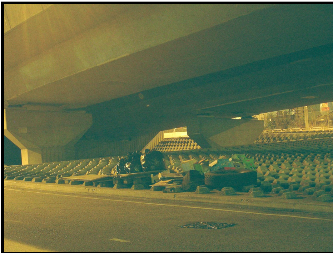
Figure 7 - Waste tyres and other trash seen under a bridge in Sham Shui Po, Hong Kong.
