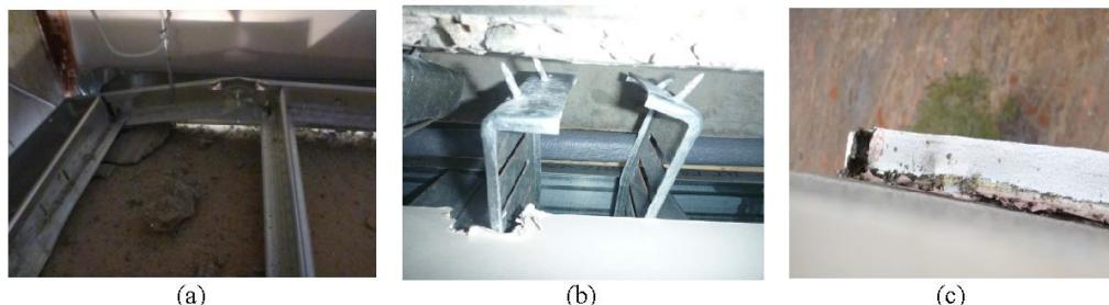
Fig. 16. Issues affecting compartment integrity (a) Gap formed at North balloon framing and ceiling joint of Floor 3; (b) detached balloon framing connection clips; (c) gaps developed at the EIFS façade.
