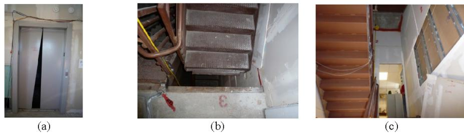
Fig. 13. Damage to egress systems following FB-6 (a) distorted elevator door on Floor 3; (b) stair detached from landing; (c) detached gypsum board around stair landing area.
