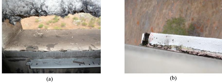
Fig. 9. Burnout of EIFS on window 4 opening (a) and smoke residue on damaged balloon framing (b)
