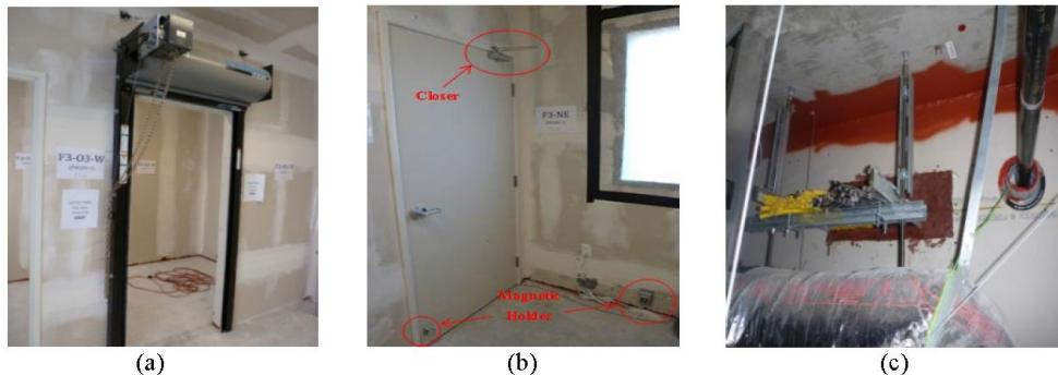
Fig. 9. Fire protection systems on Floor 3 (a) fire door; (b) door closer and holder (c) fire stop systems.
