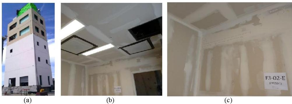
Fig. 3. (a) Façades systems; (b) Floor 3 ceiling system (c) Floor 3 partitions.
