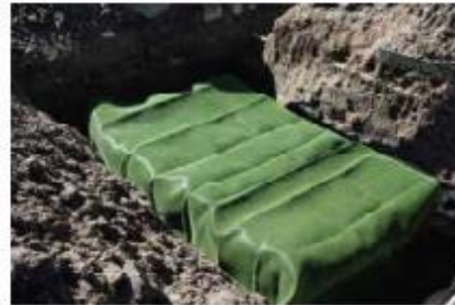
Figure 15 (Above): 12" overlap of Biaxial Mesh on top of underdrain module
