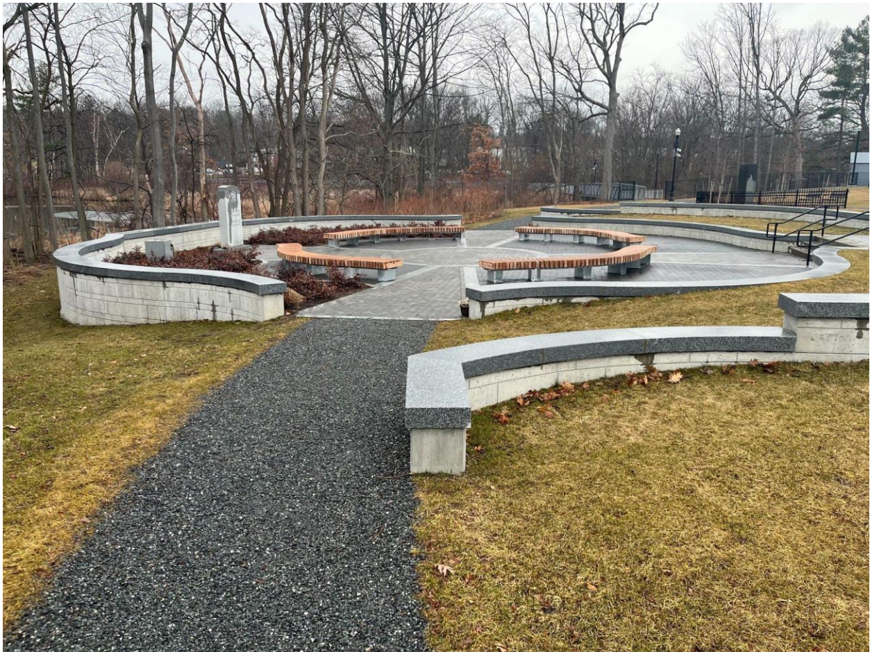
Figure 35: Rain Garden and Infiltration Walkway BMP at Worcester Fallen Firefighters Memorial
