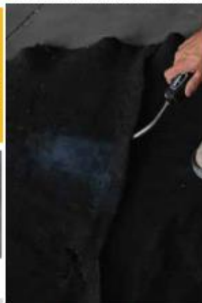
Figure 29: Geotextile being melted together with a torch.
