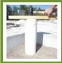
Figure 3: Hammering Pipe Into Media
