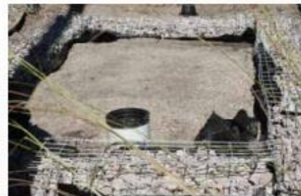
Figure 23: Level Soils once they are filled to specified depth
