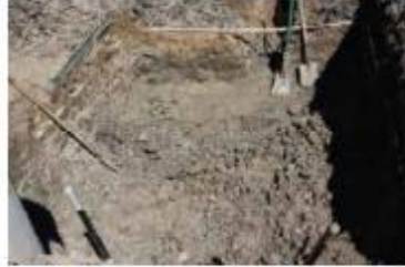
Figure 4: Excavation according to plans, following all governmental regulations
