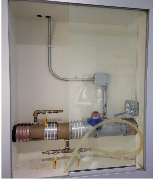
Figure 9: East Hall Green Roof Stormwater Collector
