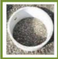
Figure 4: Pipe Installed Into Media
