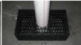
Figure 13: Place inspection port into underdrain module
