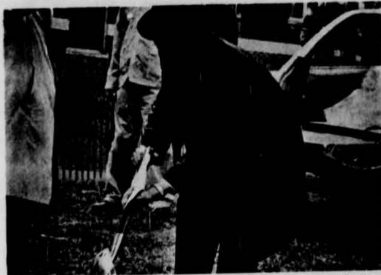
Prof. Storke breaks ground at site of new Residence Center.
