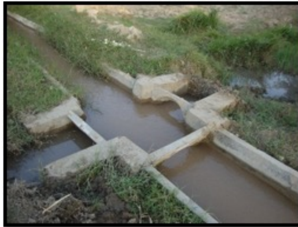
Figure 2: A channel-based surface irrigation system that distributes water by having it travel from a higher elevation to a lower one (Jamal, 2017b).
