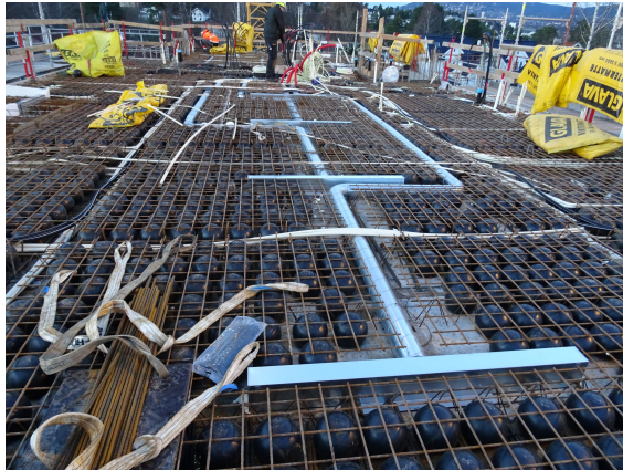
Figure 8: Precast Bubbledeck (Bubbledeck North America LLC)
