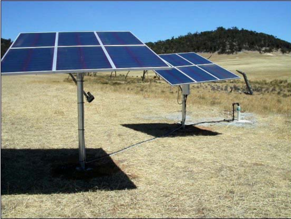
Figure 1: 720 Wp Array, ETAPUMP HR14, max. Vertical lift 42m pumping into two tanks: 1 x 1.1km, 2,000 ImpG/day , 30m vertical lift, 1 x 1.5km, 4,000 ImpG/day, 42m vertical lift . Picture Courtesy by BW Solar, Australia
