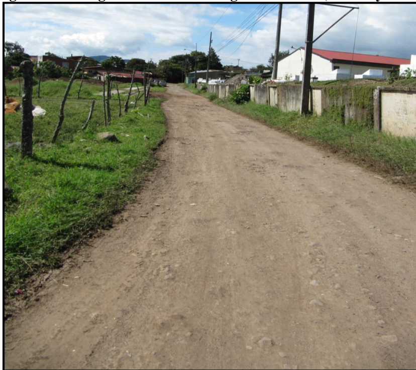
Figure 5 - Cartago site dirt road bordering Northern side (Photo by Zhang)
