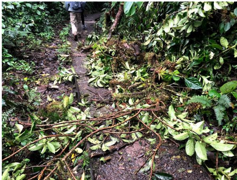
Figure A9. Fallen Branch, Encantado Main Trail
