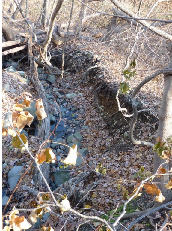
Figure 20: Eroded Runoff Channel
