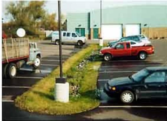
Figure 7: Vegetated Filter Strips, (Retrieved from: http://www.lakesuperiorstreams.org/stormwater/toolkit/filterstrips.html )
