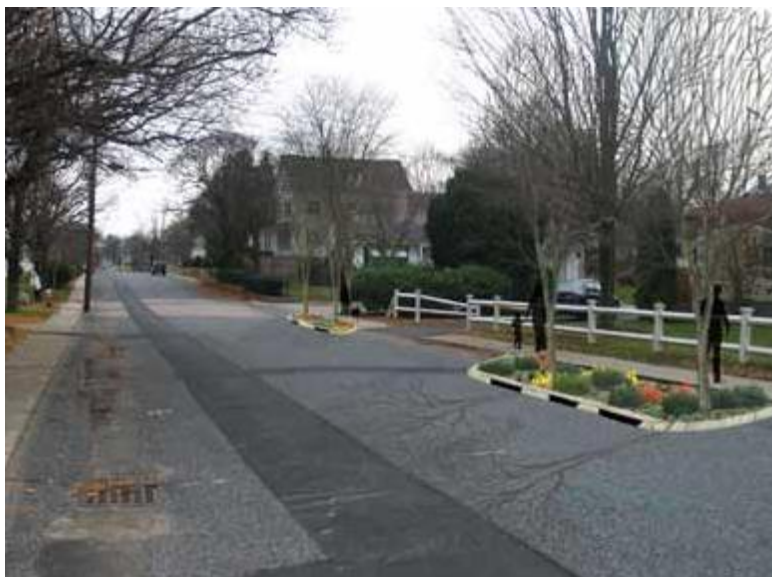
Figure 41: Bump-out Example (Image retrieved from Stormwater Management Plan for Spruce Brook Pond Subwatershed by the Charles River Watershed Association (CRWA, 2009))
