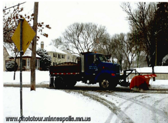
Figure 6: Snowfall, salting, and plowing accelerate crosswalk deterioration.
