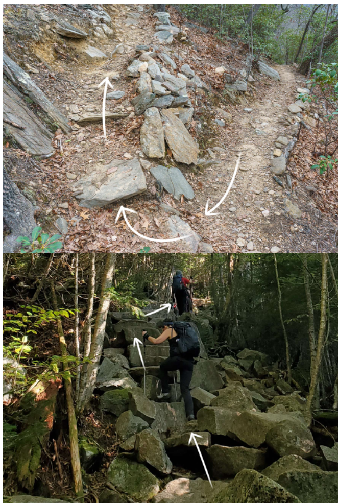
Figure 10: A comparison of two trails, a trail from a mountain in North Carolina, built with switchbacks (top). On the right is the Franconia Ridge loop trail in the WMNF which goes straight up steep rocks.
