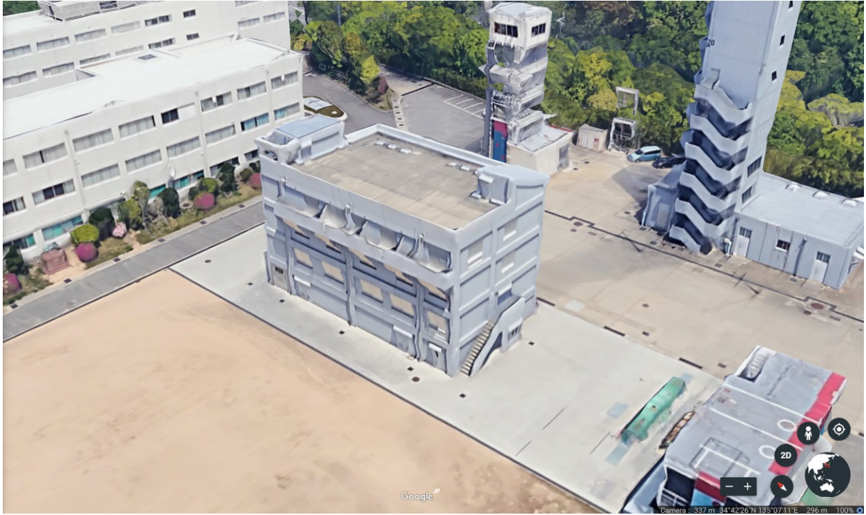
Figure 2.7: Google Earth render of the replica apartment building used for testing
