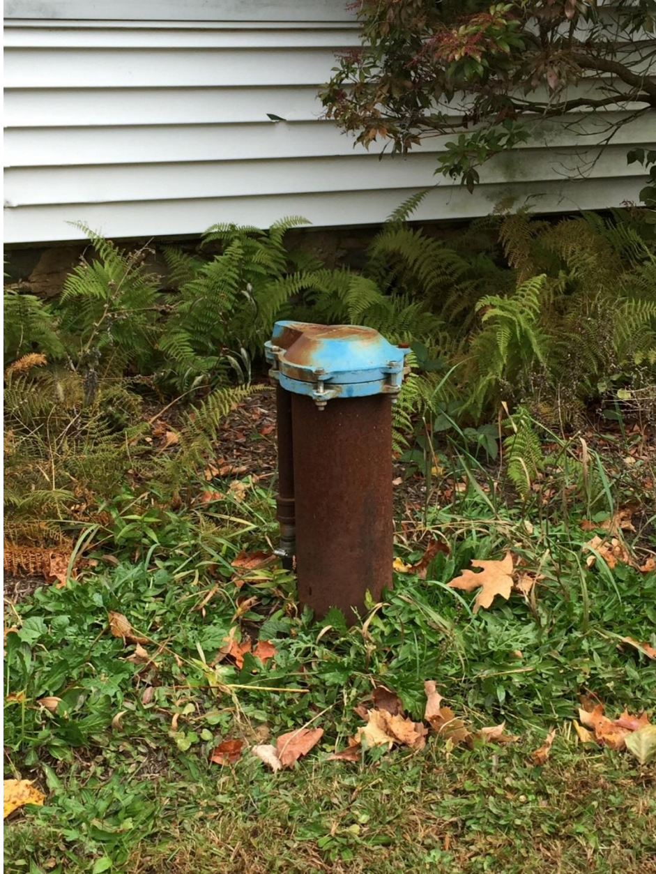
Figure 6: Farmhouse well, located next to the Farmhouse building of TVSR (GIS, 2016).
