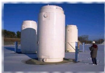
Figure 2. Dry Cask (source: thinkquest.org)
