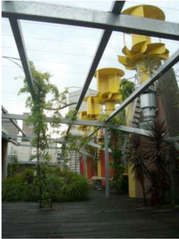
Figure 33: Rooftop of the Council House2 with wind turbines
