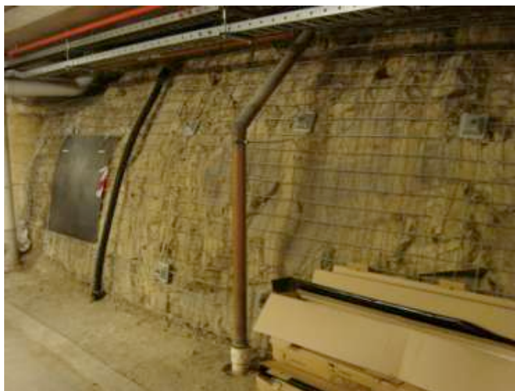
Figure 32: Rock foundation that was not blasted away; therefore, money was saved and environmental footprinting was reduced
