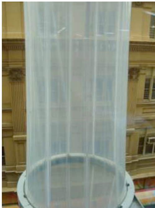
Figure 24: Rain showers that help cool the building
