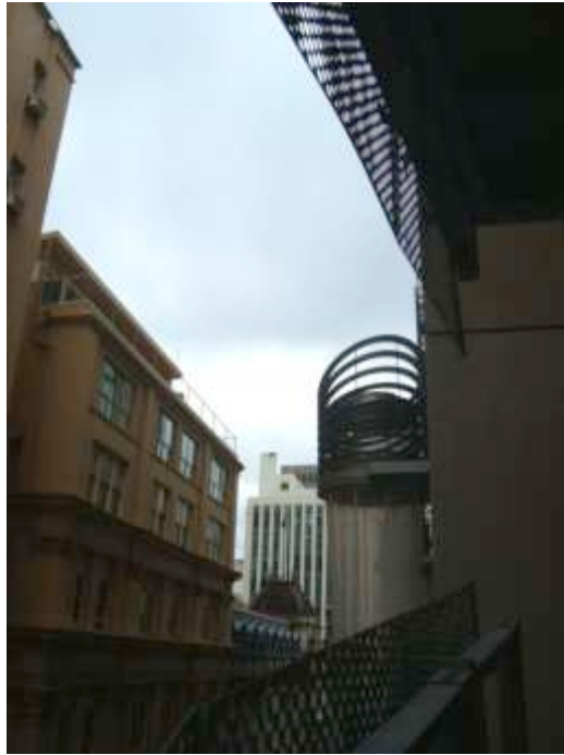
Figure 25: Outside on the deck looking at the top of the showers
