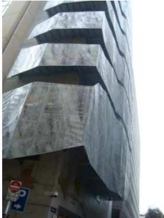
Figure 41: Overhanging toilet blocks for ventilation
