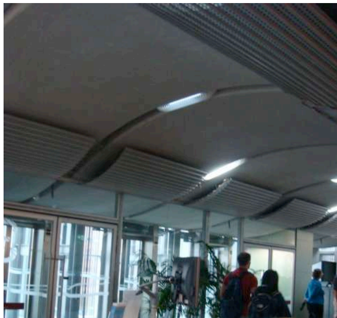
Figure 22: Lobby with curved ceilings to help air circulation and heating and cooling of the building
