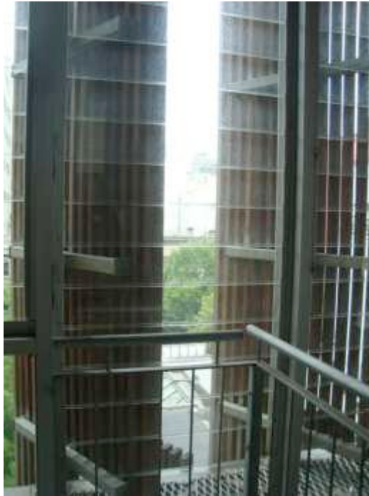
Figure 23: Shutters that adjust depending on the angle of the sun and outdoor temperature
