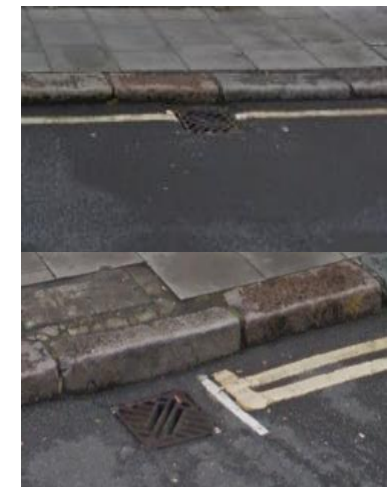
Figure 37: Gullies on Arlington Street. (Google Maps, n.d.)
