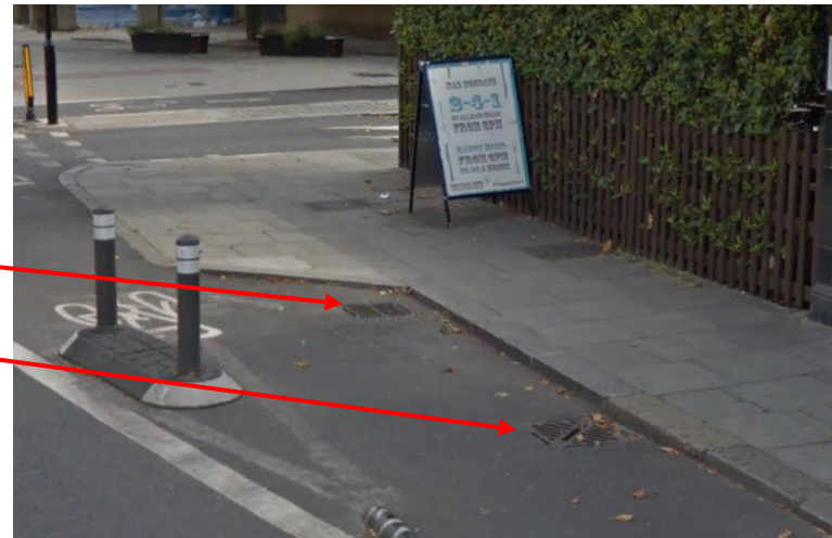
Figure 51: Gullies at the cycle lane on Royal College street. (Google Maps, n.d.)
