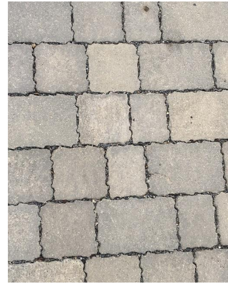
Figure 40: A photo of permeable paving.
