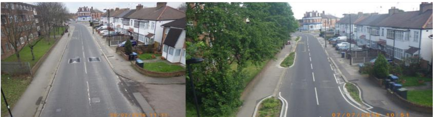
Figure 22: Comparison of Alma Road before and after implementation of rain gardens. (Mayor of London, 2016)
