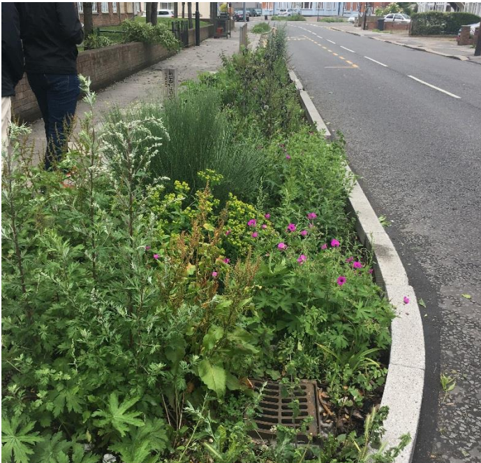
Figure 41: A photo of rain garden with a gully nearby.
