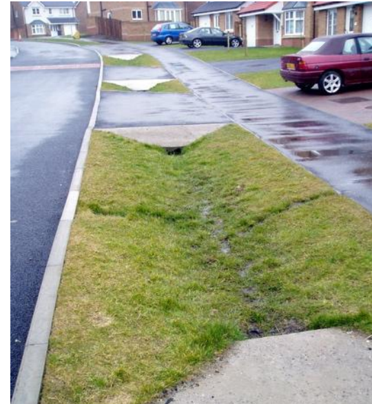
Figure 52: Example of a swale. (Susdrain, n.d.)
