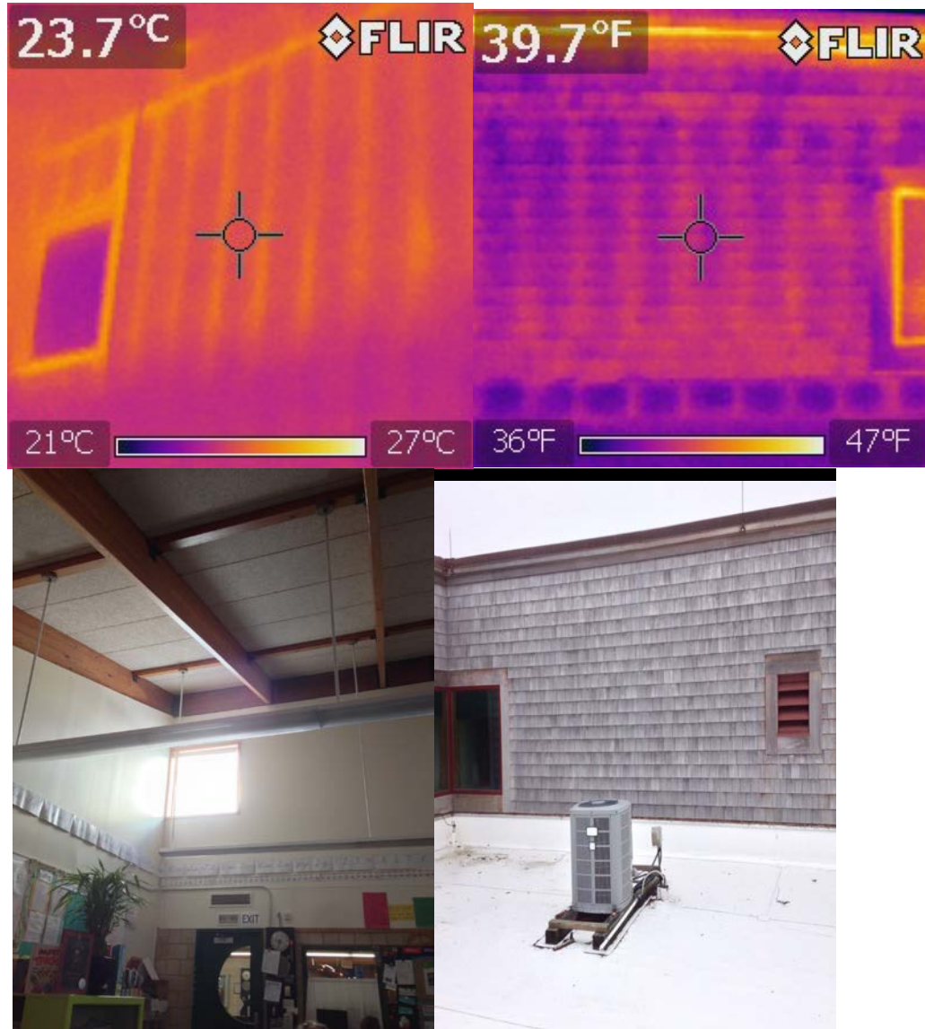
Figure 25: Internal and External FLIR Wall Photos
