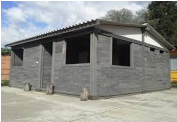
Figure 13: Plastic Brick Building- A building built through a partnership between UNICEF and Conceptos Plasticos [34]
