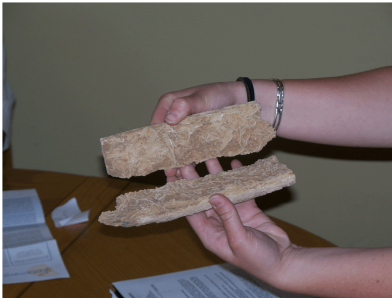
FIGURE 14: CORRODED ASBESTOS PIPE
