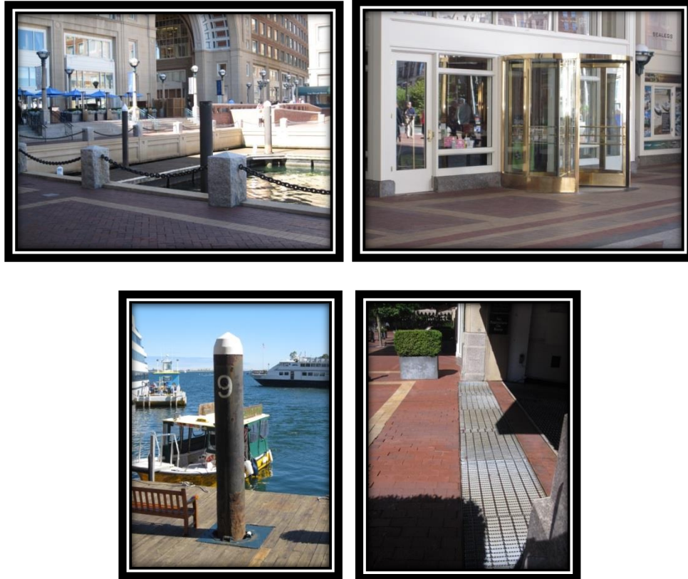
Figure 18: Pictures taken of the vulnerable features of the Rowes Wharf Complex (top left: height of seawall, top right: main entrance, bottom left: height of dock caps, bottom right: vent in front of garage)
