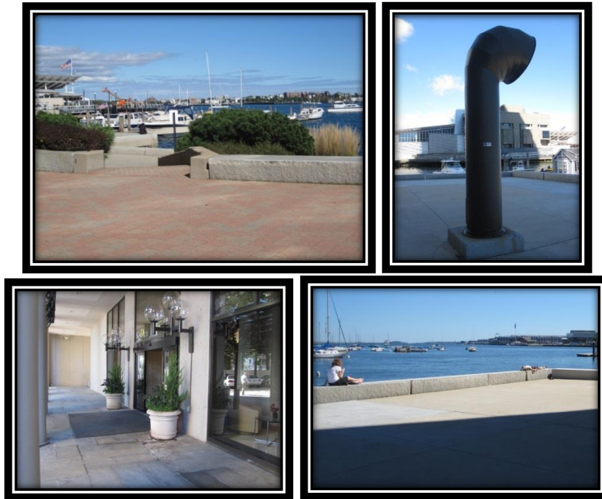
Figure 20: Pictures taken of the vulnerable features of the Harbor Towers (top left: higher seawall, top right: air vent leading to basement, bottom left: main entrance to east building, bottom right: lower seawall)
