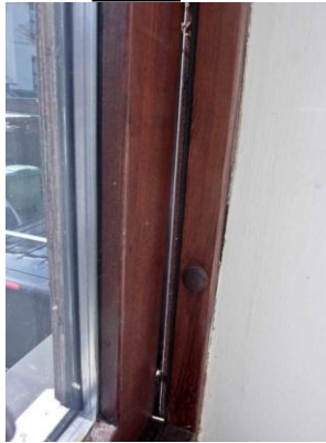
Figure 3: Warped window
