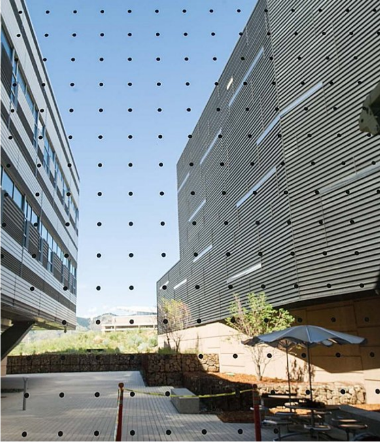
Figure 8 : This image is the exterior of a National Renewable Energy Laboratory (NREL). A dot pattern was used to help prevent bird collisions. Photo by Dennis Schroeder, featured in " Reducing bird collisions with buildings and building glass best practices ", USFWS, Public Domain
