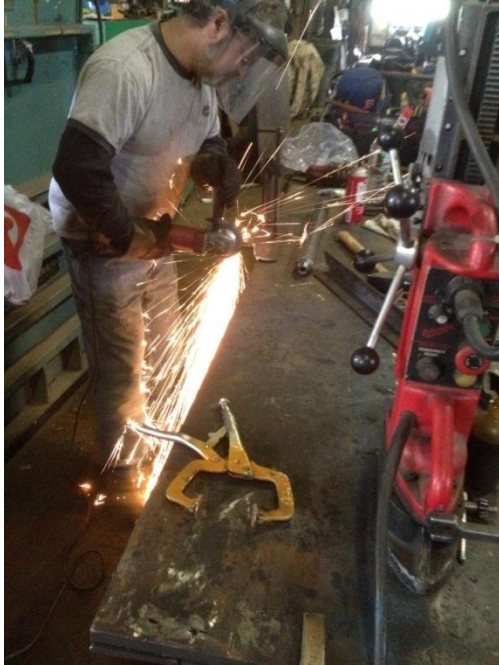
Figure 41 - Hand grinding steel plates to spec
