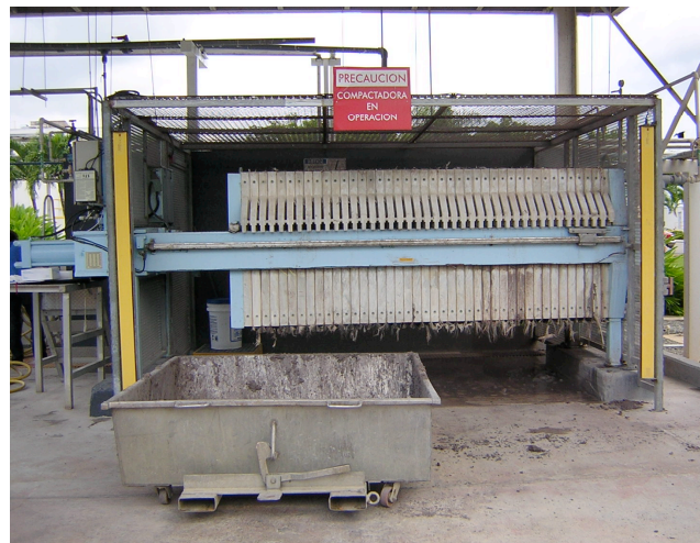
Figure 21: Plate and Frame Filter Press at Janssen Ortho LLC
