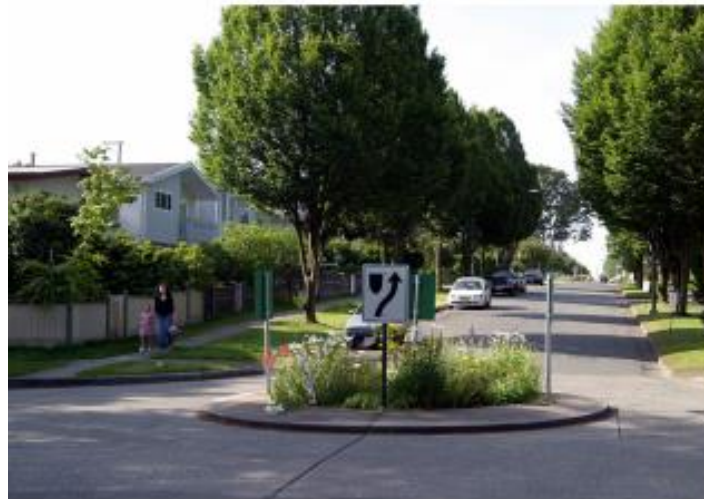
Figure 17: Mini circle in a residential area 73
