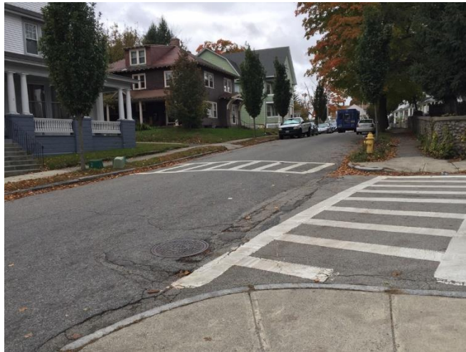
Figure 42: Lack of curb cuts on corner of Oberlin and Claremont Sq
