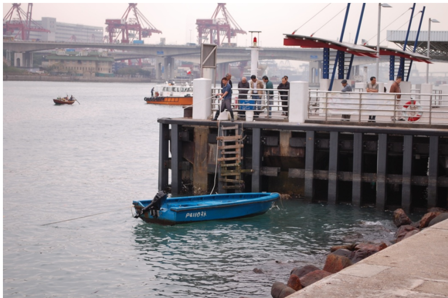
Figure 4.87: An Improvised Ladder in Tsing Yi.
