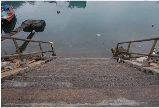
Figure 4.47: Concrete stairwell to polluted water in Lei Yue Mun typhoon shelter
