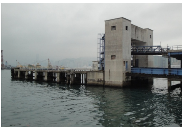
Figure 4.34: Closed off pier at Kai Tak
