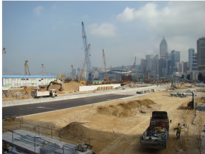
Figure 4.62: Central Reclamation Phase III
