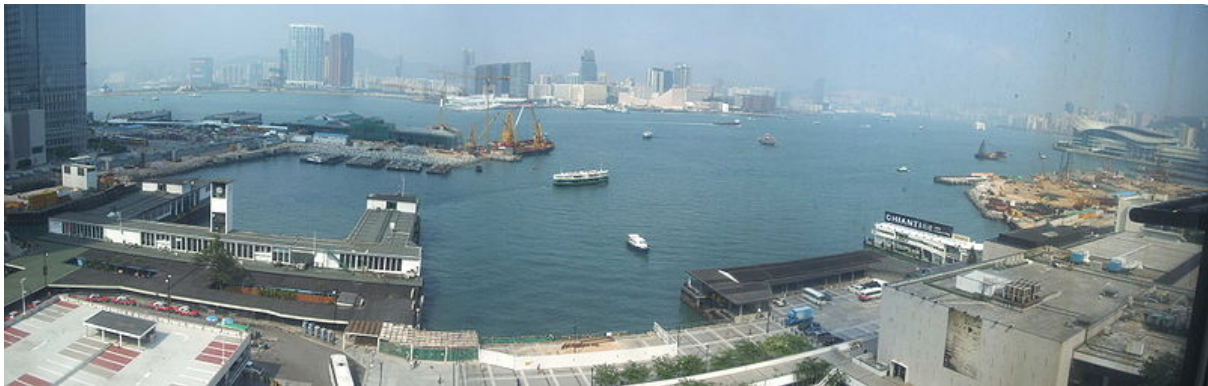
Figure 4.61: Central's waterfront, before Central Reclamation Phase III
