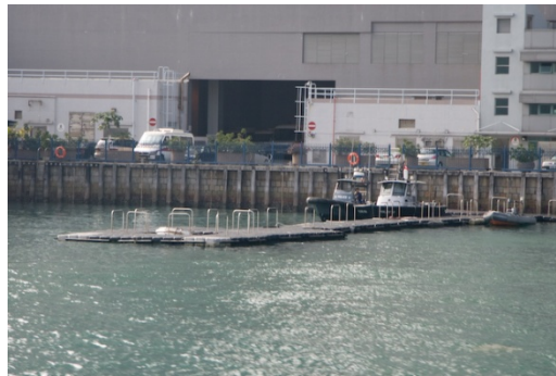
Figure 4.72: Island East marine police pier
