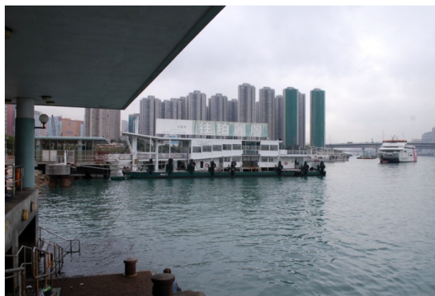
Figure 4.3: Park Island ferry terminal
