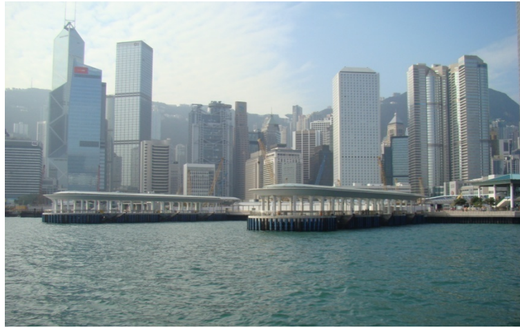
Figure 4.60: Central Piers No. 9 and 10
