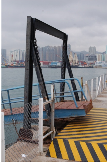
Figure 4.8: Plank hoist at Yau Ma Tei
