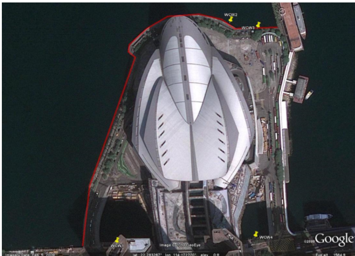
Figure 4.63: Wan Chai West
