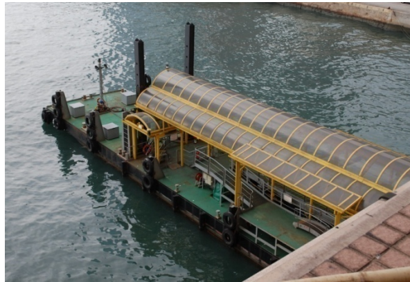
Figure 4.16: Tsim Sha Tsui West ferry floating pontoon dock
