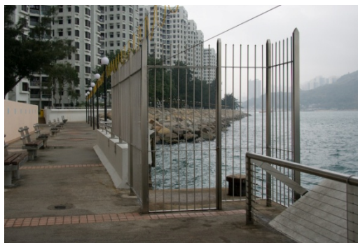
Figure 4.76: Fenced off landing step in Chai Wan
