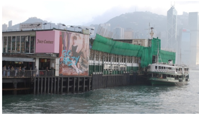
Figure 4.19: Tsim Sha Tsui East Star Ferry terminal
