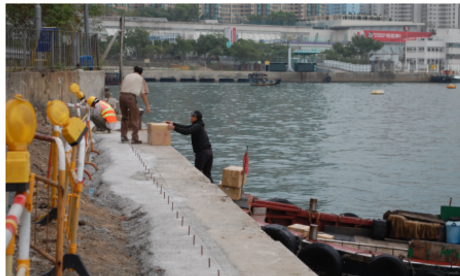
Figure 4.9: Improvised cargo-handling area in Yau Ma Tei
