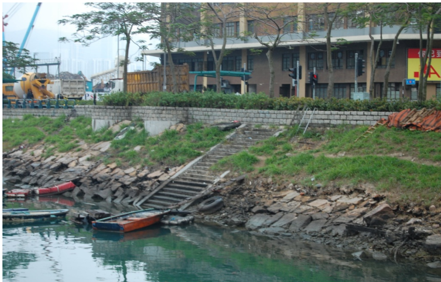
Figure 4.85: Staircase to Nowhere.
