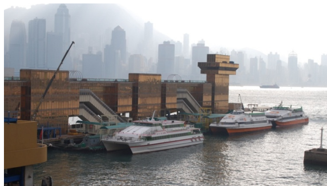
Figure 4.15: Tsim Sha Tsui West main cross-boundary ferry pier
