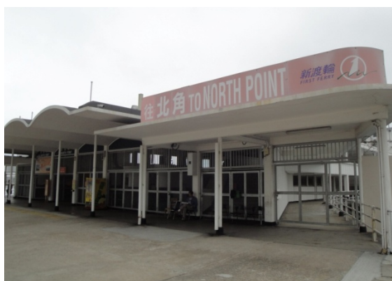
Figure 4.37: Kai Tak First Ferry terminal
