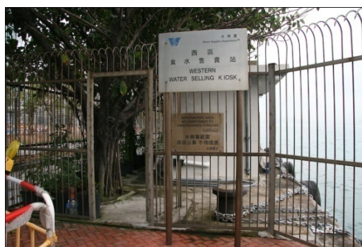
Figure 4.56: Water selling kiosk in Sai Ying Pun
