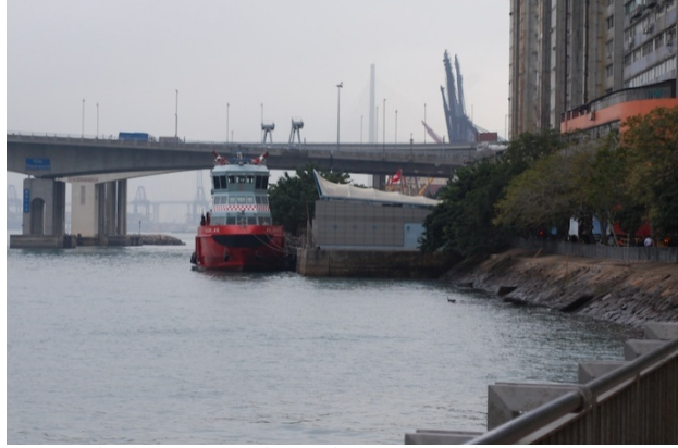
Figure 4.6: Tsing Yi fireboat fire station
