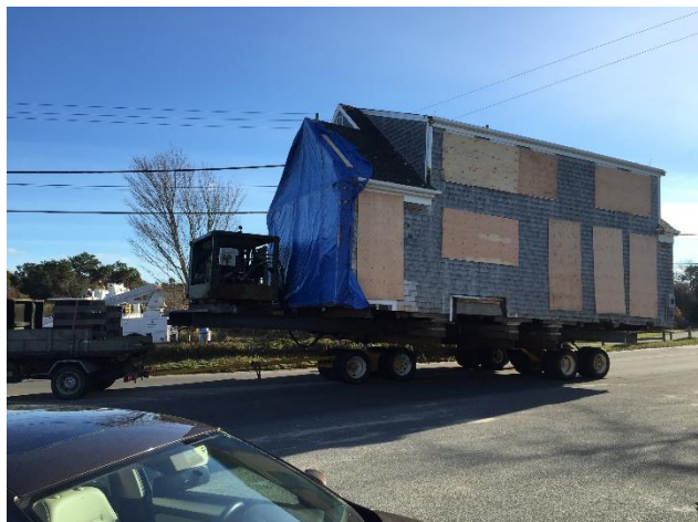
Figure 4: Example of home relocation on Nantucket
