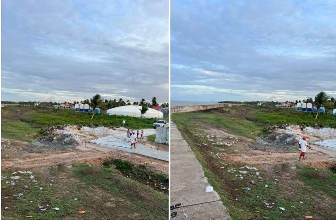
Figure 2: These images show the lot of interest from the Northwest corner. The water pump stations that are adjacent to the lot are pictured. The seawall is also pictured in this image.
